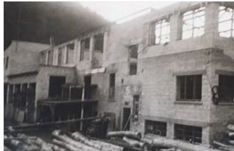
Construction of production halls for the manufacture of wooden pallets
